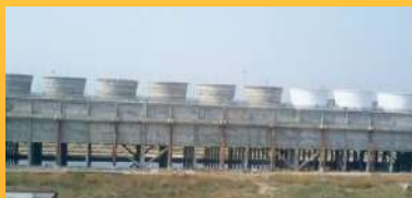
SUPER THERMAL POWER PROJECT AT NAGPUR, MAHARASHTRA
